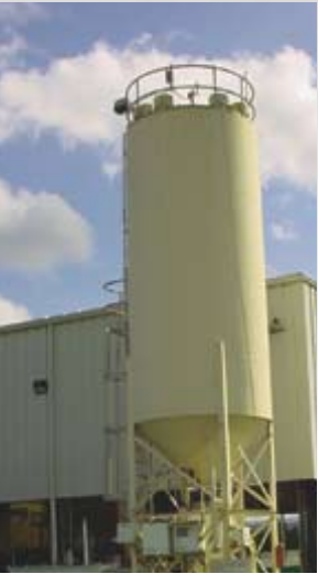
Self-contained sand silo
